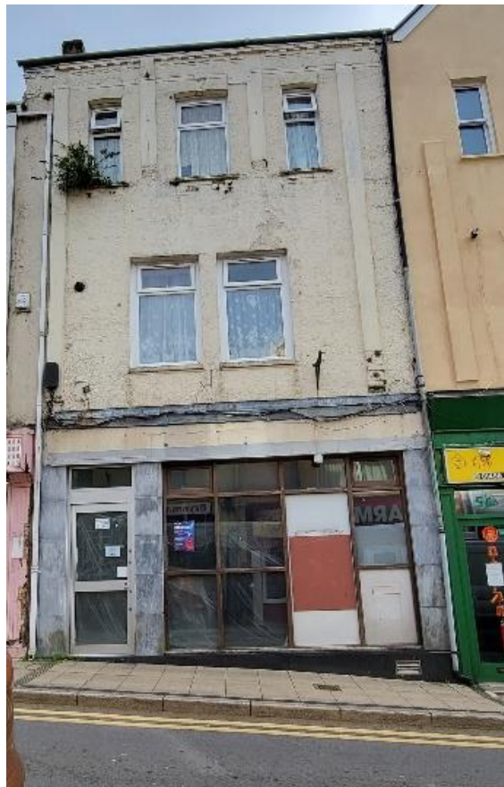
Fig. 1.1 Existing Property at 55 Beaufort Street
